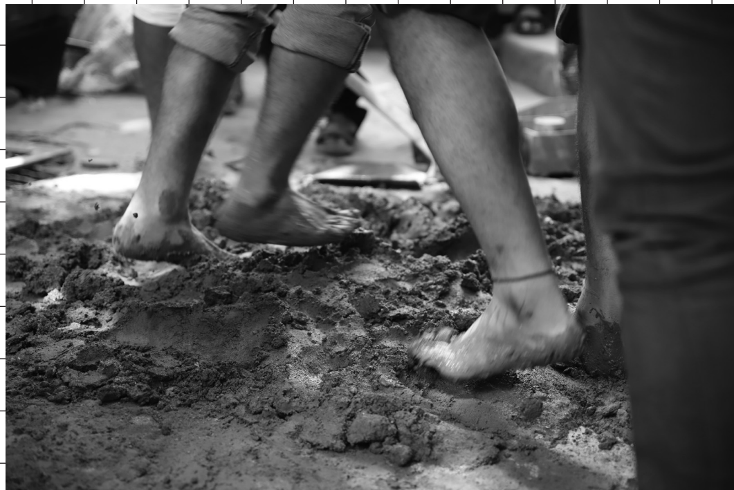
Students pugging mud at the 'Building with Stabilised Mud' workshop, July 2019, Mjinnmayee office, Bangalore. Photograph by the Curt Gambetta.
