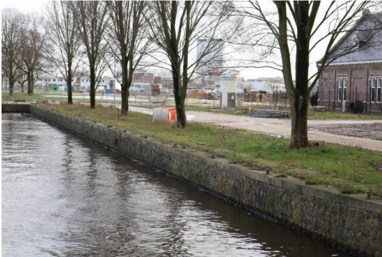
Figure 2.2, Photograph of Overamstel quay wall site to be tested.
