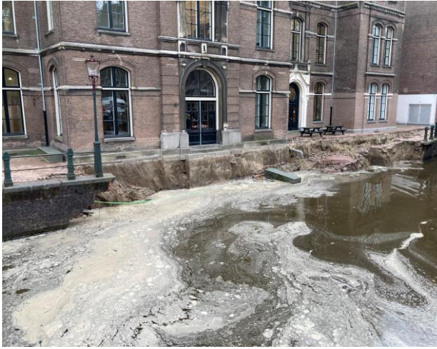
Figure 6.1, Grimburgwal directly after failure. Building in the background is the University of Amsterdam (building GB2). Left side of quay is ‘East’ and right side of quay is ‘West’. Photograph: Hugo Logtenberg, 1 September 2020.
