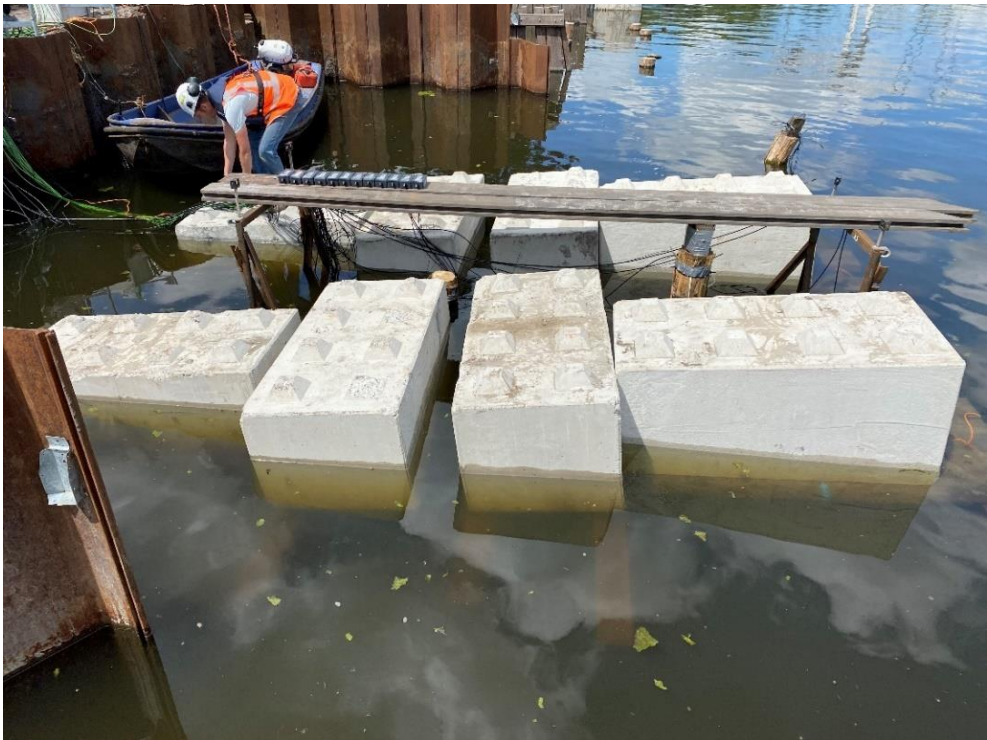
Figure 2.12, Lateral pile group experiment (3x4 pile group) with top load.
