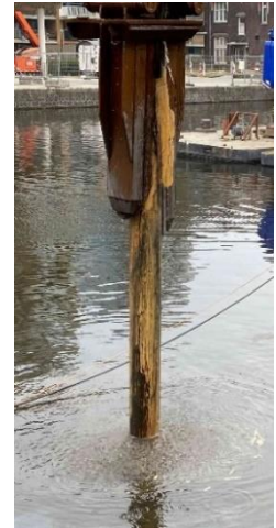
Figure 3.4, Extraction of timber foundation pile with steel pneumatic clamp under vibration.
