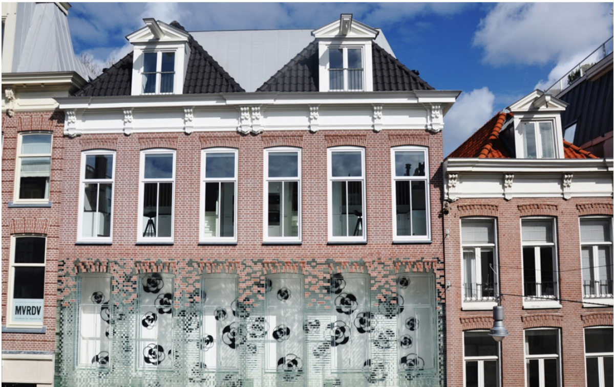
Fig. 25 End result of the intermixing, gradient zone
