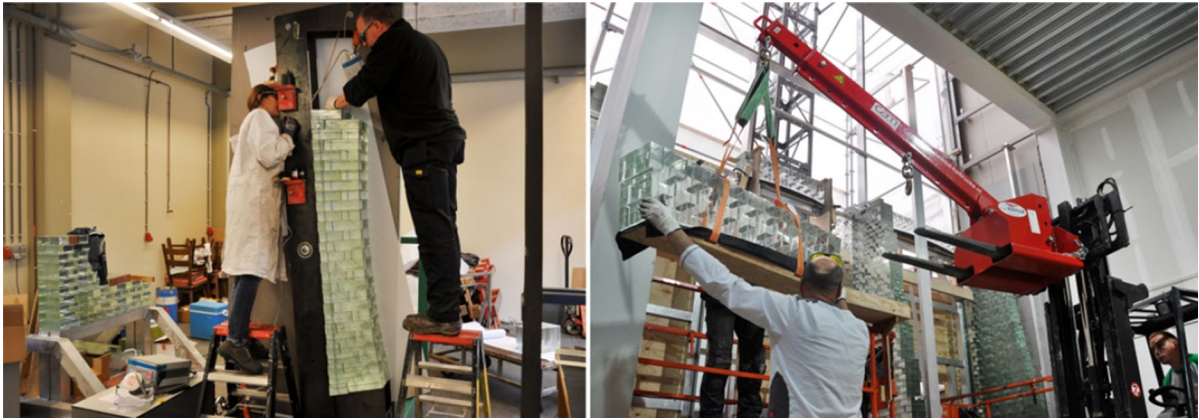
Fig. 22 Left: The special rotating fixture for the preassembly of the architraves. Right: The installation of the bonded architraves on site
