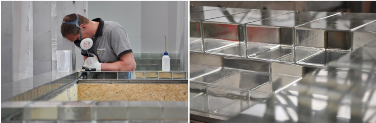
Fig. 20 Left: Sealing of the already bonded bricks. Right: the final, visual result achieved by the novel bonding method
