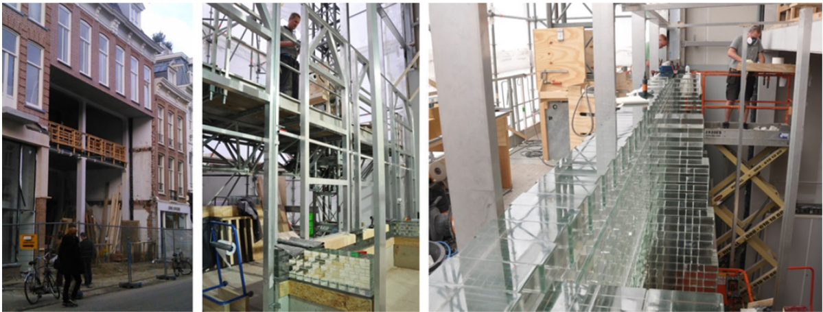
Fig. 14 Left: The masonry wall was already constructed prior to the glass elevation. Centre: the installed aluminium place holders of the opening. Right: The mast climbing working platform and one of the three mobile elevated platforms
