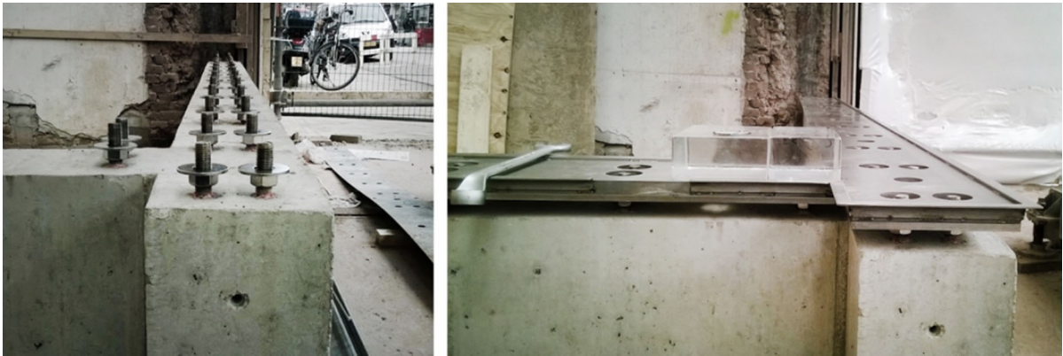
Fig. 15 On the left the bolts used for levelling the stainless steel plate, seen on the right
