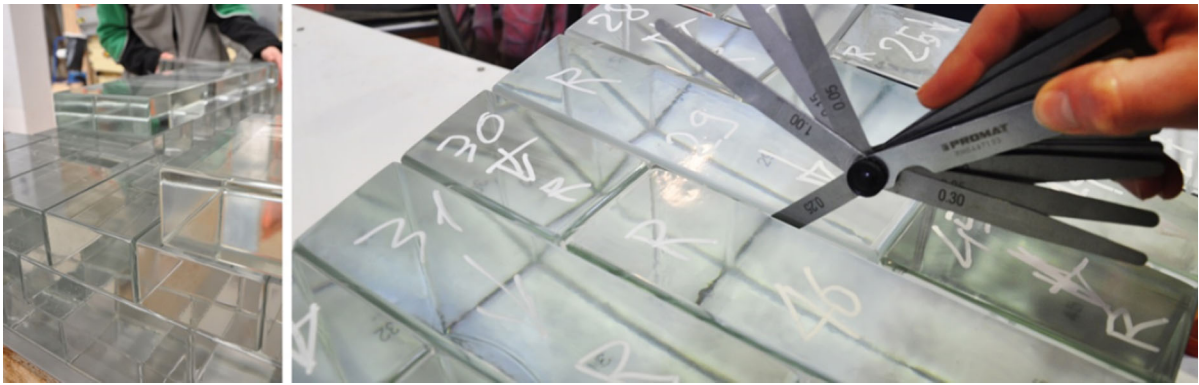
Fig. 17 Bricks of a new row laid down prior to bonding ( left ). Then a feeler gauge is used for checking the thickness of the resulting seam ( right ). The blade of the feeler gauge is sufficiently flexible and round not to induce any surface damage on glass
