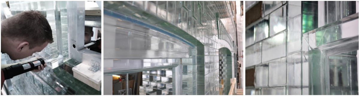
Fig. 28 Left: The simultaneous application of the polymer from both sides. Centre and right: The final result of the bonded glass frames
