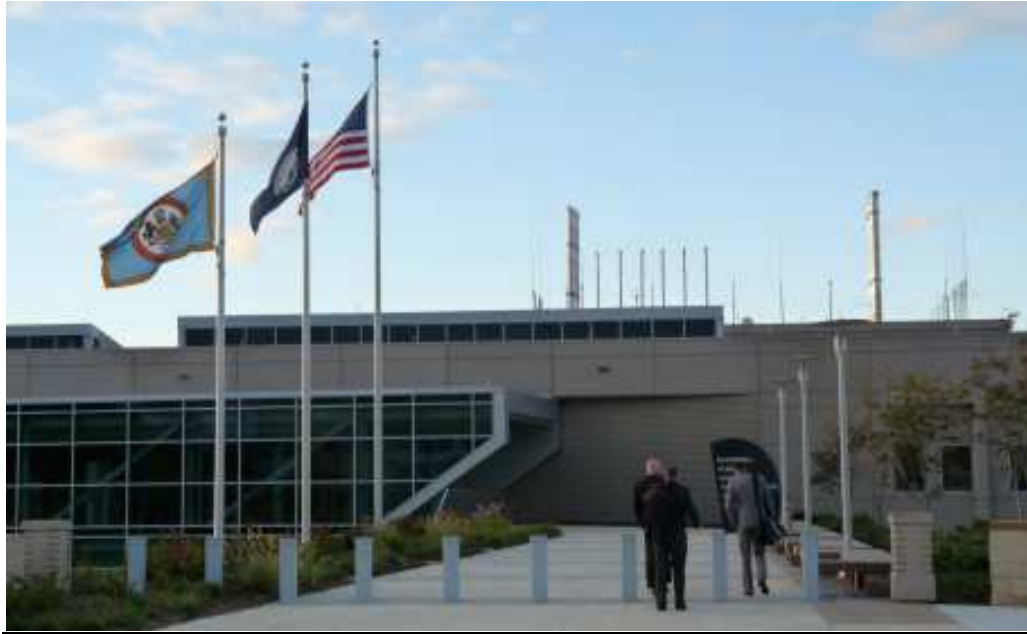
Figure 7: McConnell Public Safety and Transportation Operations Center
