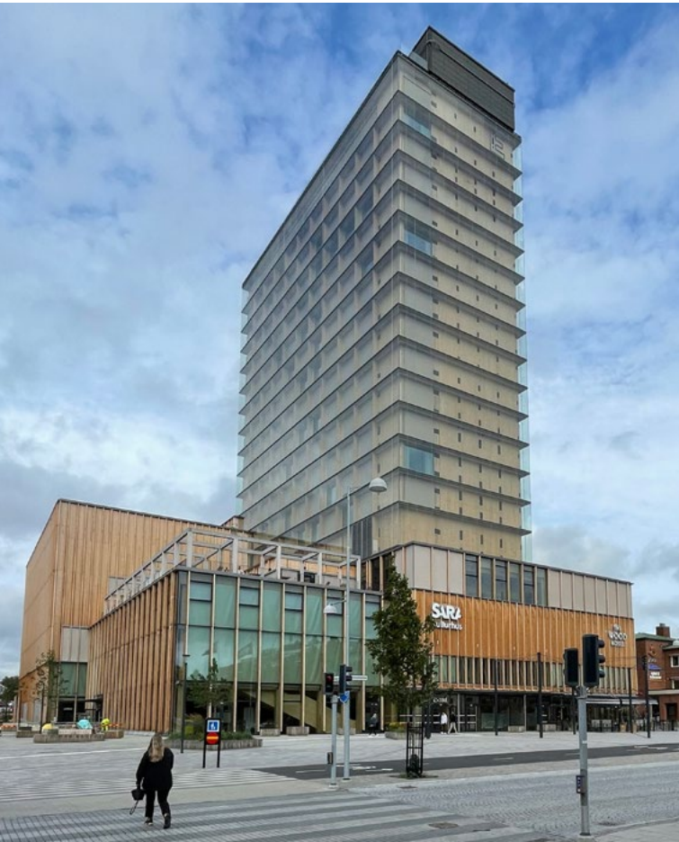
Fully wooden high-rise building, Sara Kulturhus, Skellefteå (SE), a culture centre with theatre, library, conference halls, and hotel (White Arkitekter).
