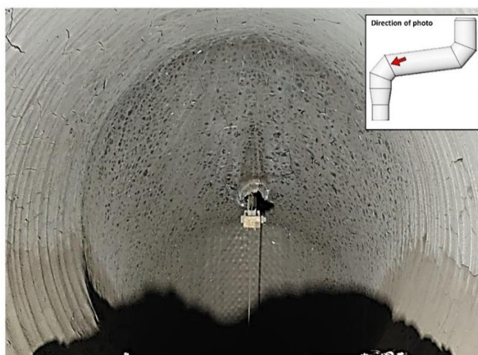
Figure 5-9. Wall condition around the oxygen lance and first bend of the dog-leg geometry (inspection 2019)
