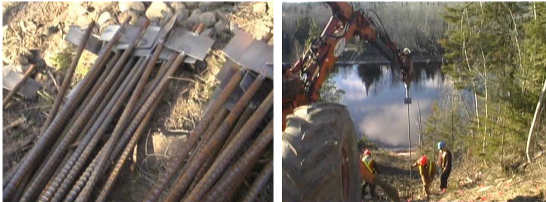
Figure 19: Left: Soil nails of 35 mm with a plate for extra resistance against shallow soil flow. These were used to stabilize a 30 m high riverbank along the Kaministiquia river in Canada, with nails in a grid of 1 m to 1.5 m. Right: nails were installed using percussing hammering (Fabius et al., 2008).
