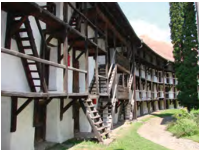
Refuge castle, Prejmer, 1220-1870, courtyard
