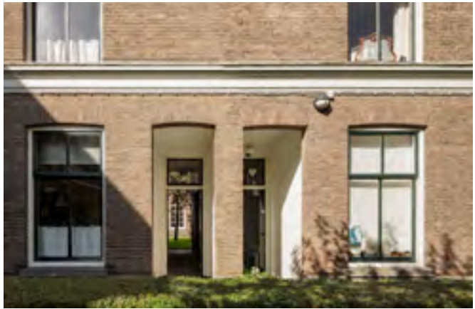
Passage between Achterhof and Langehof
