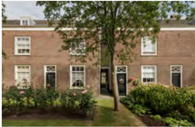
Passage between Langehof and Achterhof
