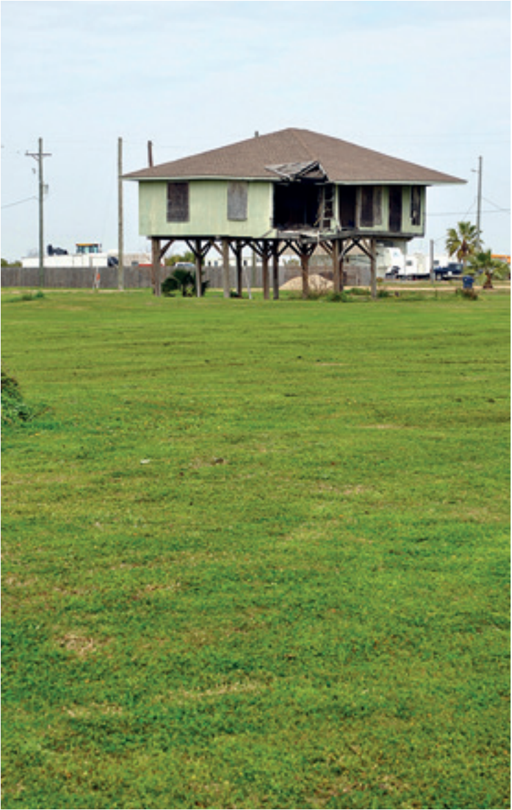
Figure 2. Elevated but still destroyed residence at Galveston Island, never repaired after Hurricane Ike (Photo courtesy Helena Van Boxtelaere).
