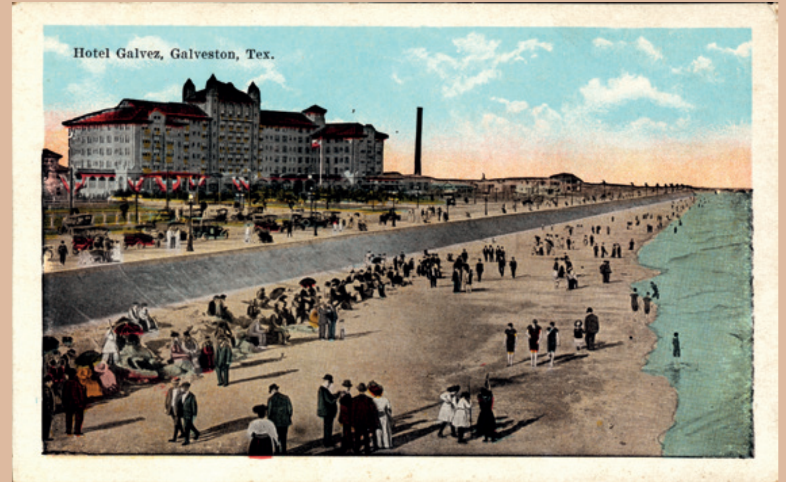
Figure 1. Multifunctional use of flood protection structures is not strange to Texas. The Galveston Seawall, here depicted on a postcard dating from 1911, was built with a road and hotels on top, as a response to the 1900 Great Hurricane (image courtesy University of Houston Digital Library).
