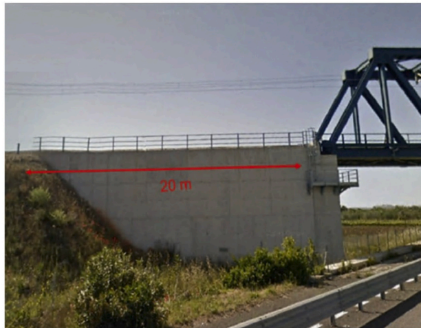
a.1 Wing walls
