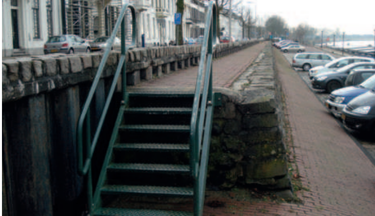
Figure 1. MFFD Zutphen, parking area in- tegrated in flood defense (photo courtesy Mark Voorendt).
