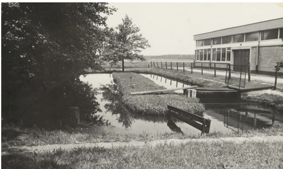
Figure 1.1: First oxidation ditch ('oxydatiesloot' in Dutch) in the Netherlands by the design of A. Pasveer in the town of Voorschoten, commissioned in 1954. It was decommissioned when the neighborhood 'Dobbewijk' (400 population equivalents) was connected to the main sewer networks and the centralized wastewater treatment system in 1996(!). Courtesy of the Rijnland District Water Control Board.
