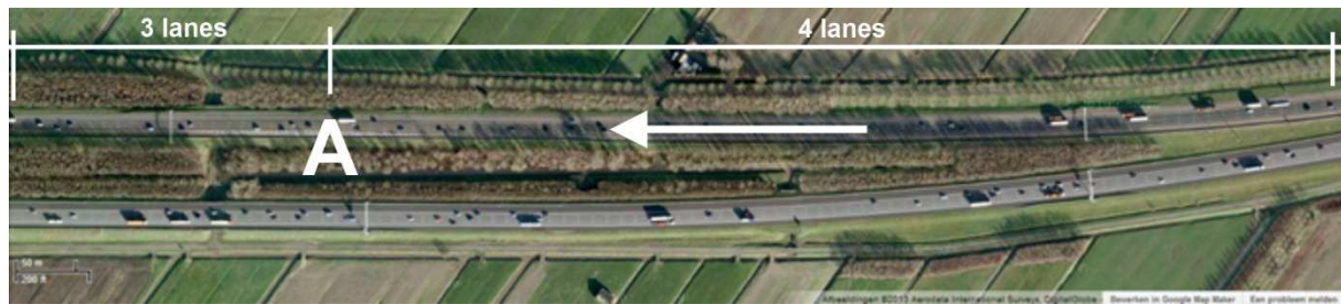
Figure 3 Bottleneck location near Woerden at the considered road section on the A12 used in the case study
