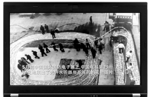
Figure 5.34 Left: Cable perpetration of the underwater Sound Surveillance System (SOSUS) hydrophone seabed array. Still from "Watch in the Sea: Project Caesar", Navy and Marine Corps Productions 24458-DN, c. 1960. Right: Cable perpetration of the 'Underwater Great Wall' fiber-optic hydrophone array. Still from "China has begun to build the 'Underwater Great Wall', and the whereabouts of uninvited guests are under control!", China Central Television (CCTV), 24 May, 2018. http://military.cctv.com/2018/05/24/ARTID2GKodHKQivW8tinDka4180524.shtml
