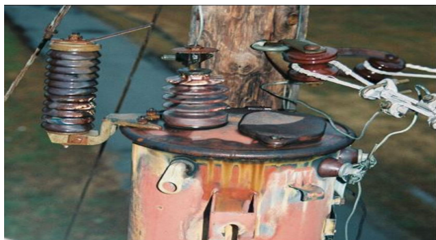
FIGURE 12. Damaged external bushing that caused intermittent faults [3].
