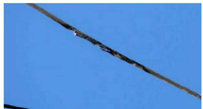
FIGURE 10. Conductor damage from wind-induced conductor slap [3].
