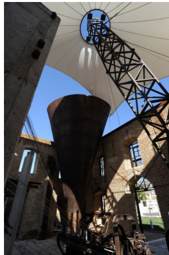
Textile museum, after adaptive reuse; addition of a horn in the center of the building in memory of the horn that existed in this factory according to one of the old employees ( https://rb.gy/fzatpe )
