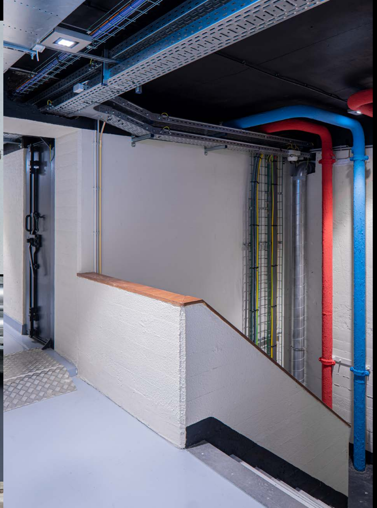
↖ Transformers transform high voltage 10kV to 400V. ← Ducts and air conditioners on the exterior wall, for cooling the servers and to air-condition the former command and control room. ↑ The painted red and blue tubes connect to the super chillers and are part of the cooling system of the Databunker.
