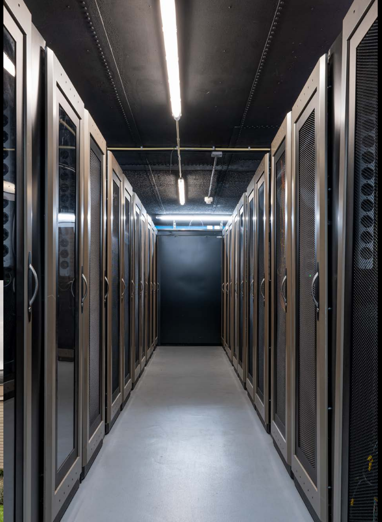
← Entrance with solar panel array and ram raid barriers. ↑ A 'hot corridor' in one of the co-location rooms, containing server racks under a black steel ceiling.
