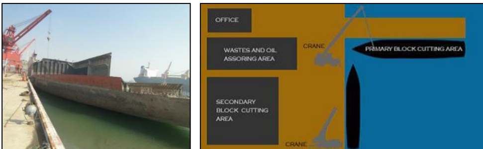
Figure 2.8: Left – A ship docked alongside for recycling (Source: Author’s personal visit to a ship recycling yard in China), Right – Pictorial representation of the alongside method (Lee, 2012)
