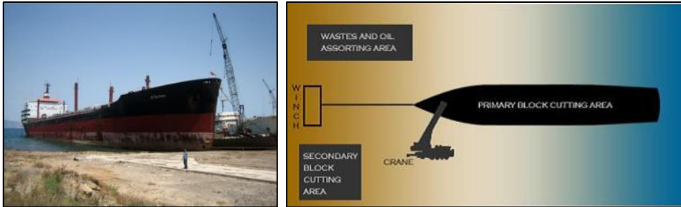
Figure 2.7: Left – An EOL ship beached at a Turkish recycling yard on a slipway (Vardar, 2009), Right – Pictorial representation of the slipway method (Lee, 2012)
