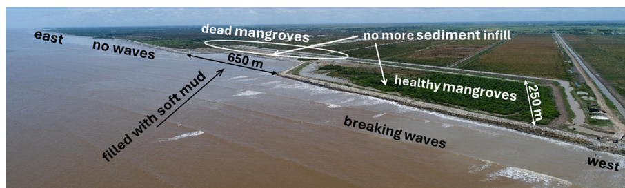
Fig. 12. Mud infill into Danzig Bay, mudflat development and mangrove colonization (drone image of September 22, 2022).
