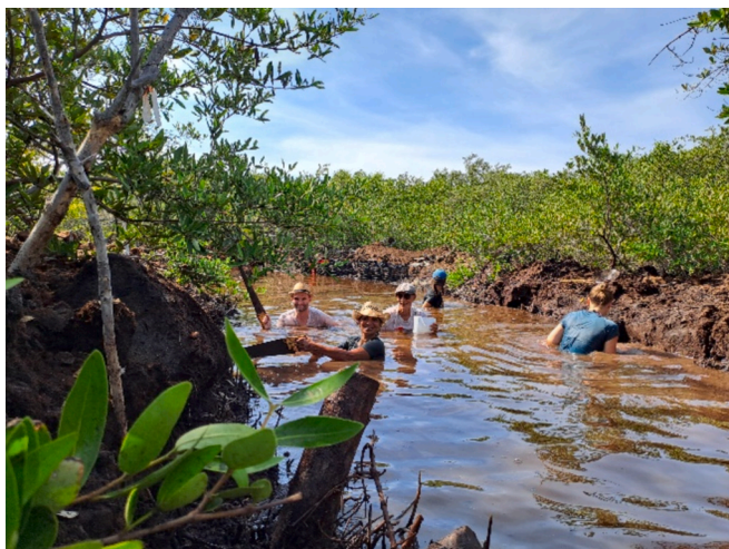
Fig. 4. Re-opening drainage channels in mangrove forest.
