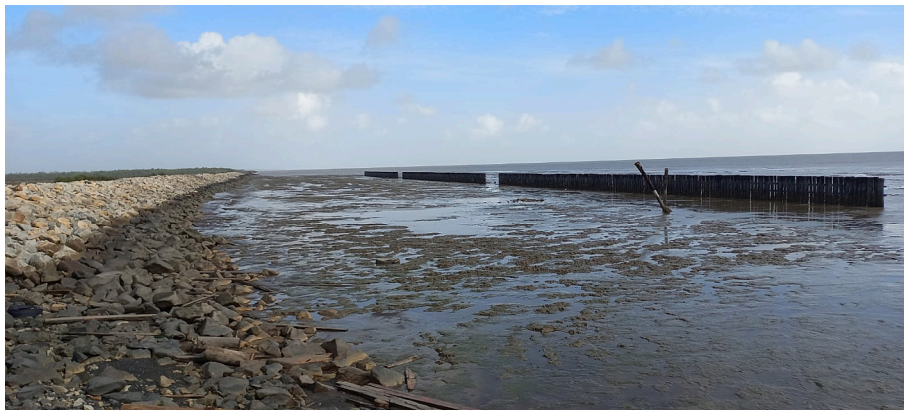
Fig. 7. Detached pile-groin breakwater at de Hoop, constructed in 2023.
