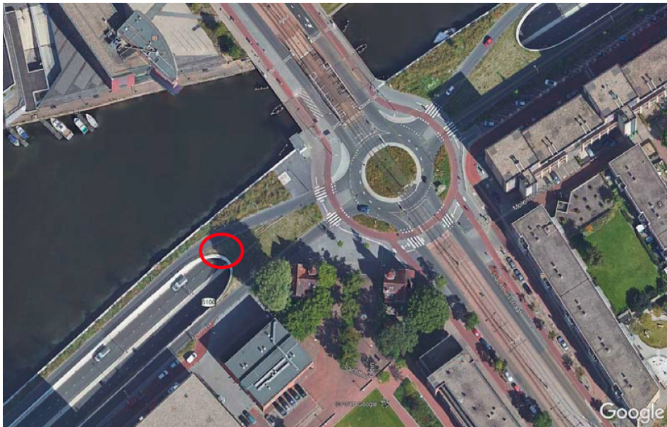
Figure B2.9: Location and orientation of underpass Neherkade, The Hague. Source: Google Maps
