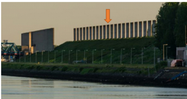
Wind deflecting structure Caland channel
