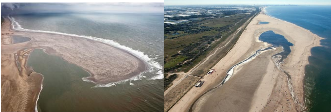
Figure 1. Aerial photographs of the Sand Engine a) just after construction in (September 2011) and b) five years later (September 2016). Photos by Rijkswaterstaat/Joop van Houdt.
