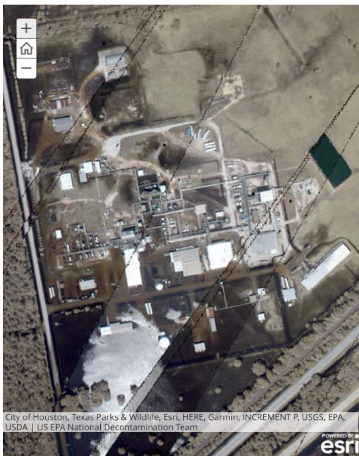
Figure 5.3. The EPA states on their Response to Hurricane Harvey: “Arkema Facility, Crosby TX. At the Arkema chemical plant in Crosby, emergency responders undertook a 24-hour operation to monitor the facility due to fires that erupted on August 31 and September 1, 2017.” (Text and image retrieved from epa.gov.arcgis.com ; October 17, 2017).
