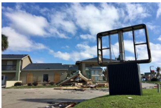
Figure 2.4. (a) Damages in Rockport, Texas were primarily wind and surge driven, whereas (b) damages in Houston were driven by extreme precipitation. (Images courtesy of (a) FEMA - Dominick Del Vecchio and (b) www.defense.gov)
