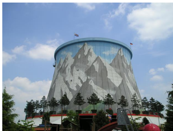
Figure 7.3: Example of re-use of concrete structure: former cooling tower of nuclear power station Kalkar (Germany): nowadays a climbing wall as part of the amusement park (source: www.Wikipedia.org )
