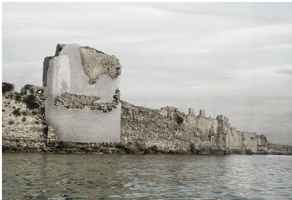
Figure 1. Illustration of the cast glass masonry
