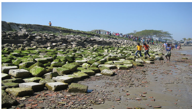
Figure 2.10. An eroded Dyke on the Island of Bhola, Bangladesh. Retrieved from https://www.royalhaskoningdhv.com/nl-nl/nederland/nieuws/nieuwsberichten/20140625pb-nl-experts-ontwikkelen-kustbeschermingsplan-bangladesh/3333
