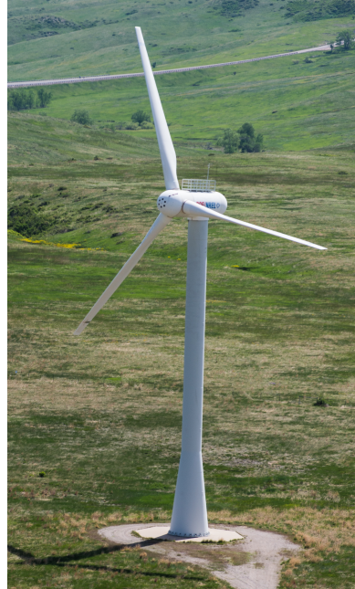
(b) This figure is showing the 600 kW Controls Advanced Research Turbine (CART) III wind turbine in Colorado, United States of America. Photo by Dennis Schroeder, NREL 37892.
