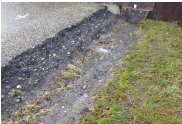
Fig. 3 Damaged transition present before the experiment in Millingen aan de Rijn started (Bakker et al. 2013). The damaged grass sod highly influenced erosion development on the landside transition
