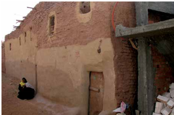
FIGURE 2.22 Concrete frame construction replacing load bearing walls, Dakhla oasis, Egypt
