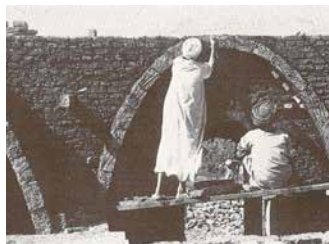
FIGURE 2.19 Building traditional vaults using clay bricks in Egypt
