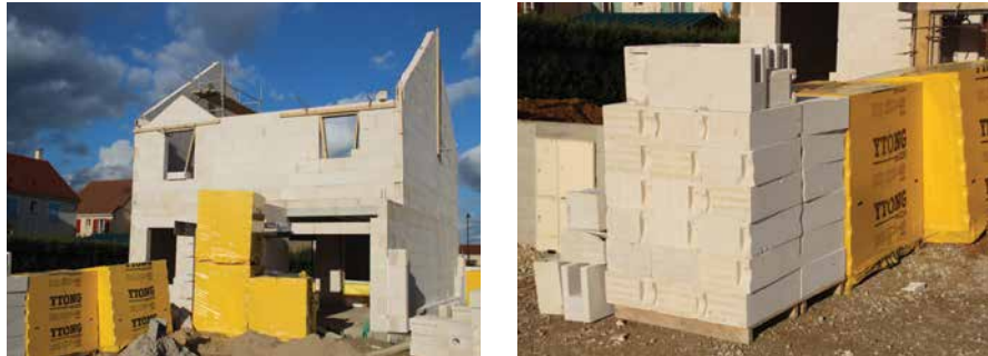
FIGURE 5.31 Ytong blocks at a project site
