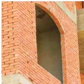
FIGURE 6.1 A 12-cm thick external walls found in many current constructions
