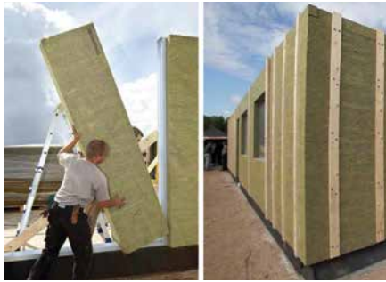
FIGURE 1.1 Insulation panels providing load-bearing function
