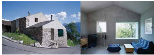
FIGURE 4.15 Renovation of Roduit House in Chamoson, Switzerland using Expanded Glass Concrete
