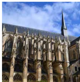
FIGURE 2.12 Flying Buttresses of Abbaye de la Trinité, France
