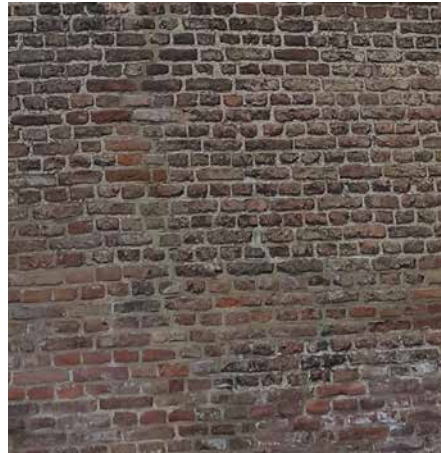
FIGURE 2.5 The brick pattern of the Old Church in Delft
