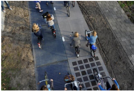
Fig. 5. Estimated Operating Efficiency of the Solar Road in Year 2015, estimated dc power output in the same year and installed Solarroads in the bike lane in the village of Krommenie, North Holland [12].
