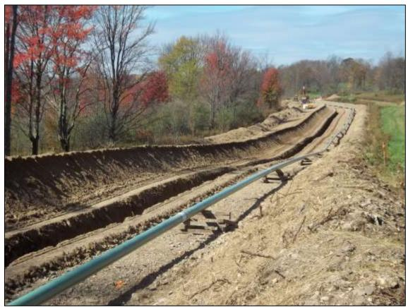
Figure Y-63: NEPA pipeline trenching (lindeco.com).
