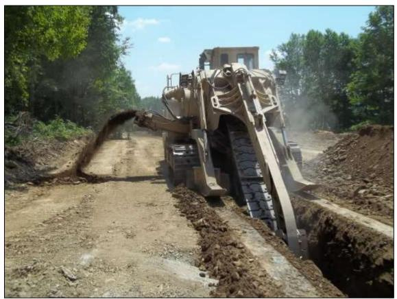
Figure Y-62: NEPA pipeline trenching (lindeco.com).
