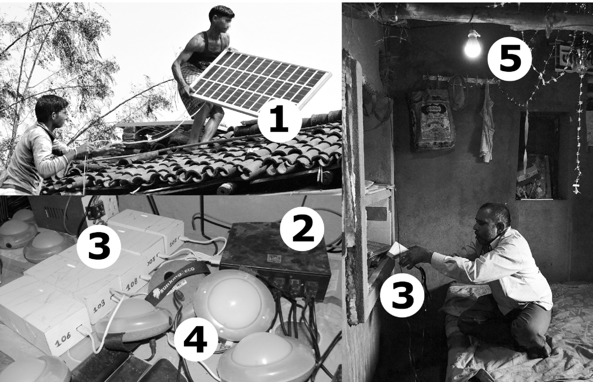
Fig. 4. Energy Distribution Infrastructure. Note the labels: '1': Solar Panel; '2': Energy Router; '3': Power banks; '4': Solar Lantern; '5': LED Bulb.
