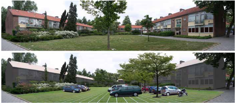
FIGURE 8.5 Above: existing semi-public inner courtyard. Underneath: Adaptation measures which improve thermal comfort and increase parking space are light roofs, middle-dark facades, additional trees and permeable pavement with grass.
