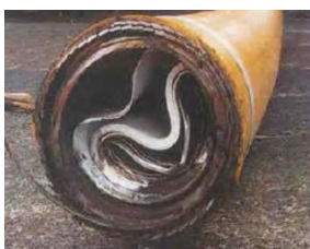
Figure 2. Collapse failure of the flexible riser [7]
