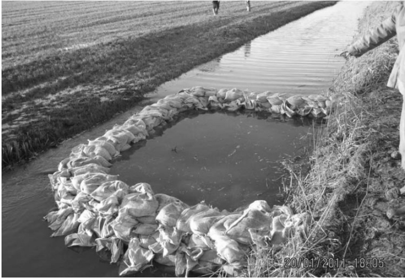
Figure 16: Sandbags to prevent piping during the high water in the year 2011 [Source: Waterschap Rivierenland]
