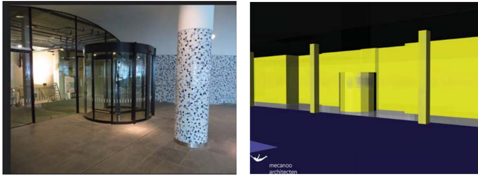
Figure 11. Revolving door of the municipality of Delft extending into the property of another party.
