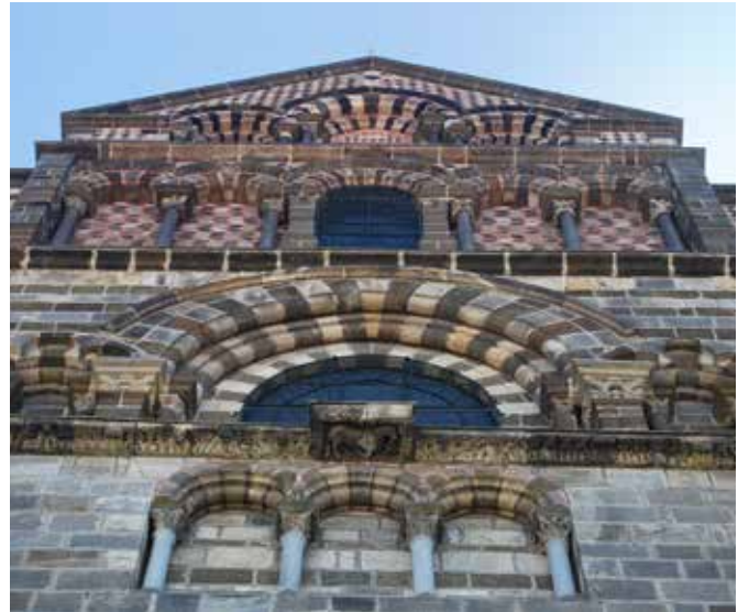
FIG. 3.26 The upper part of the façade of the Notre Dame de Puy-en-Velay, where skin and structure are inseparable / Marieke Kuipers
