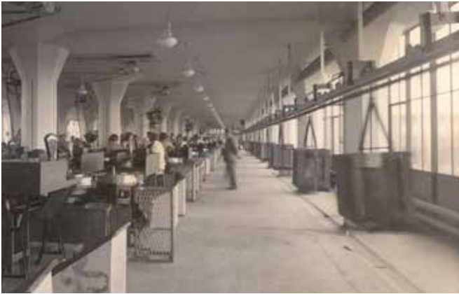
FIG. 2.11 The interior of the Van Nelle Factory in the late 1920s, featuring novel light fixtures and a conveyor system / Jan Kamman – Gemeente Archief Rotterdam
