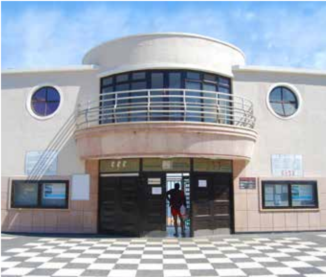
FIG. 3.25 The entrance pavilion of the Sea Point swimming pool, Cape Town / Marieke Kuipers
