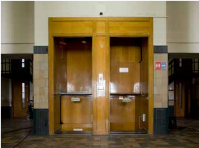
FIG. 3.41 A paternoster lift in former Post Office, Rotterdam / courtesy of the Cultural Heritage Agency of the Netherlands
