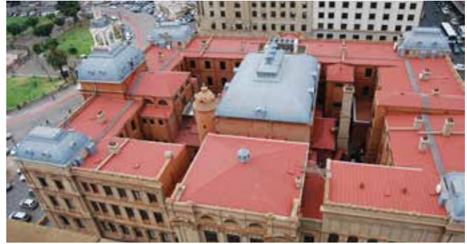
FIG. 3.21 The roof of the administrative buildings of Old Raadsaal by the Dutch-born architect Sytze Wierda located on Church Square, Pretoria / Marieke Kuipers
