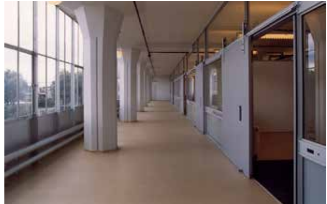
FIG. 5.28 A view inside the double-skin façade at the eastern side, where the cavity doubles as a corridor, required for proper circulation in any case / Fas Keuzenkamp, Pijnacker
