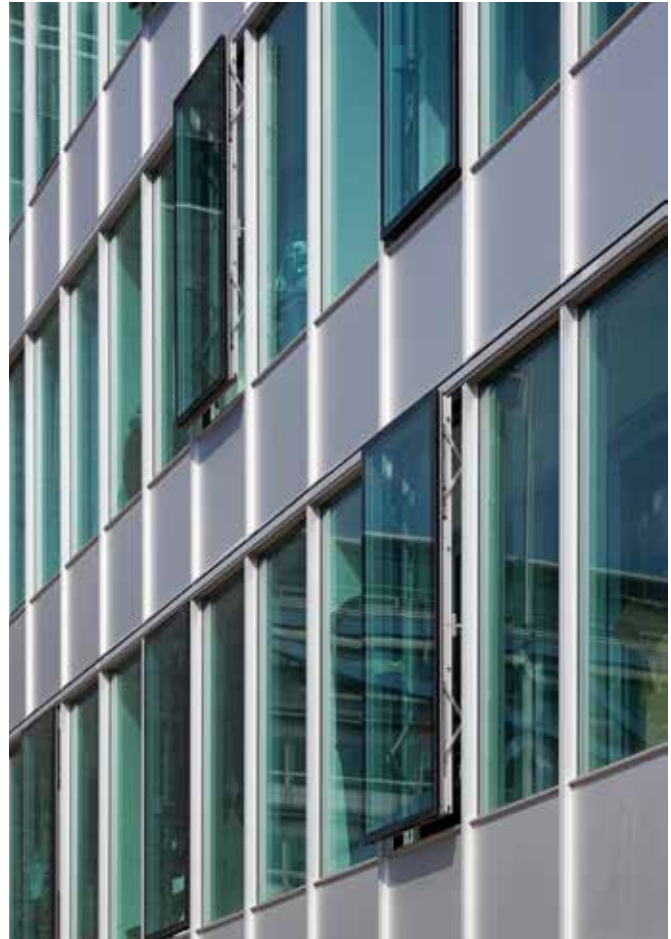
FIG. 5.36 Close up of the redesigned new façade after replacement around 2015, featuring operable windows that project horizontally outward / Luuk Kramer
