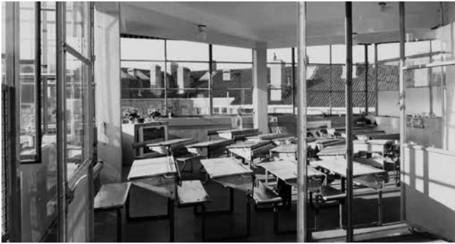
FIG. 5.30 Duiker understood that the only way to heat the (largely) open-air class rooms was to rely on radiation; he had heating pipes embedded in the reinforced concrete floors to make them act as radiation panels / W. J. van Berselen, Stadsarchief Amsterdam
