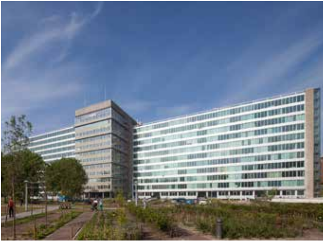
FIG. 2.27 The GAK Building in Amsterdam in 2015, after its transformation into housing for young professionals / Luuk Kramer
