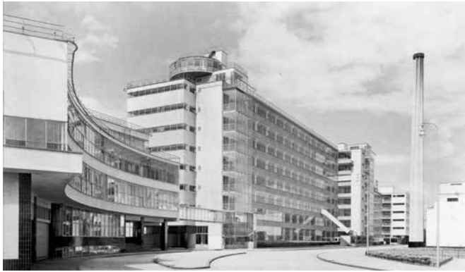
FIG. 2.6 The Van Nelle Factory as seen from the entrance in 1930 / Evert van Ojen – Gemeente Archief
