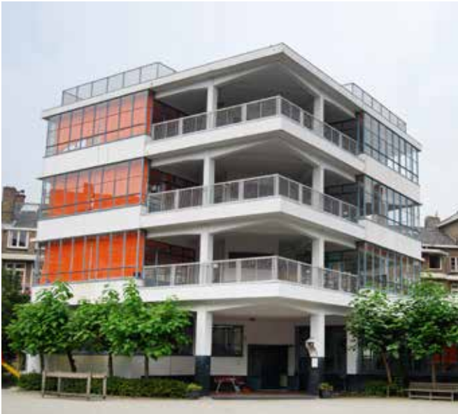
FIG. 3.9 The Amsterdam Open Air School, designed by Jan Duiker, with loggias deliberately orientated southwards and a rooftop that was originally intended for lessons in the open air, weather permitting / Marieke Kuipers
