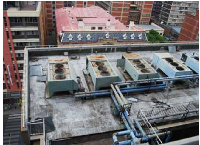
FIG. 3.40 Architecturally integrated air conditioning systems in the former TPA Building, Pretoria / Marieke Kuipers
