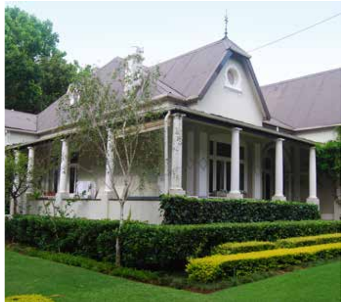
FIG. 3.10 Typical 'stoeep' or veranda surrounding a house in Pretoria provides outdoor space in shade / Marieke Kuipers
