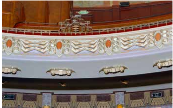
FIG. 4.13 The restored cinema hall of the Art Deco Tuschinski theatre at Amsterdam (originally built in 1921), with murals by Pieter den Besten (recently restored) and new emergency exit light / photo: courtesy of the Cultural Heritage Agency of the Netherlands
