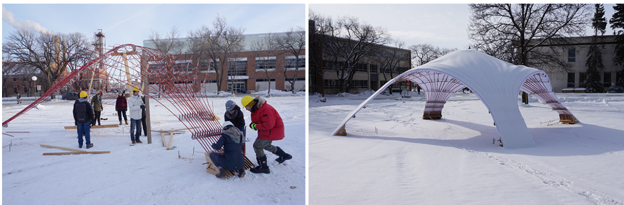
Figure 1: Students assembling the bending active framed vault (left), completed ice shell structure (right). [photos by Dominique Rey & Lancelot Coar]
