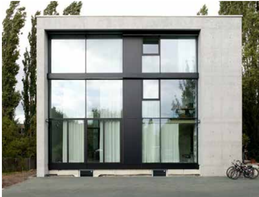
FIG. 1 Single family home with outer ILC walls in Berlin, 2007 (Photo: M. Schlaich)
