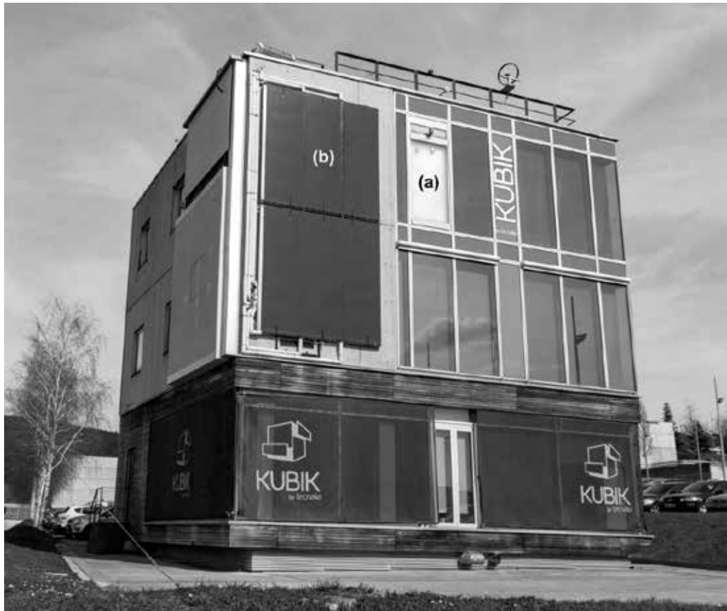
FIG. 5 Pilot set-ups at south-facing façade of KUBIK test facility: (a) integrated solar air collector (RETROKIT, 2016), (b) hybridized sandwich-type steel envelope (BASSE, 2016)
