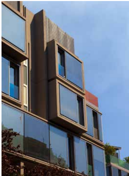
FIG. 6 To further emphasize the image of the all-glass effect at the corners or the openings, the outer slab of the insulating glazing extends 10-15 cm beyond the inner slab to cover the rising.
