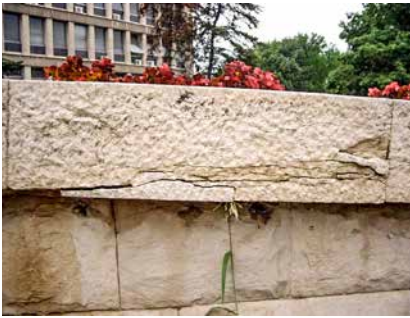
FIG. 2.1 Marble damaged by the effects of low temperatures (Stefanović, 2010)
