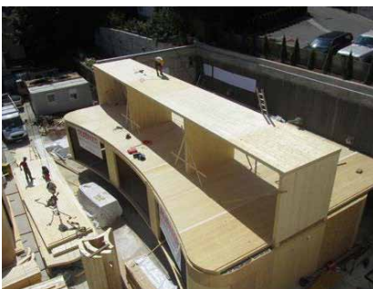
FIG. 3.3 From the left: Prefabricated CLT elements are transported to the construction site and then assembled and erected manually – Waldorf School in Ljubljana, Slovenia.
