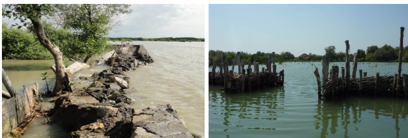
Fig. 9: Erosion near coastal revetment Indonesia (left) and Building with Nature pilot for mangrove development (Demak, Indonesia, right)
