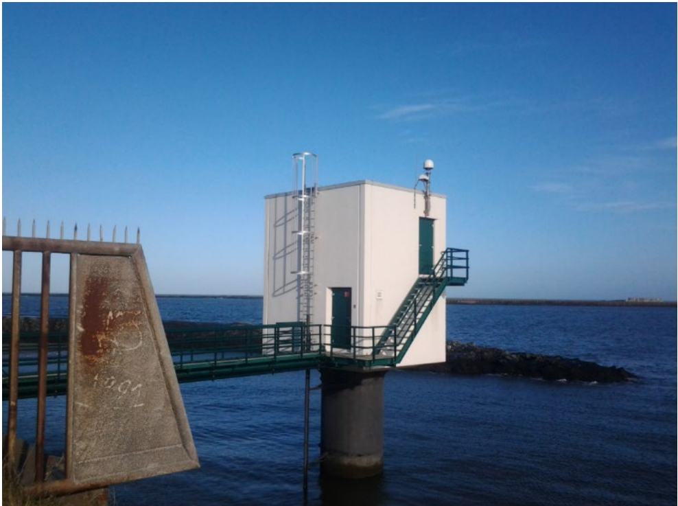
Figure 4-4: LMW Measurement Station (RWS, 2017)
