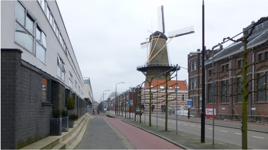
Figure A.8: Improved Noordendijk, Dordrecht, March 2013 (river side at the right)
