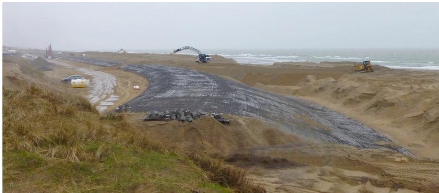
Figure 6.9: Katwijk: construction of the dike-in-dune, February 2014
