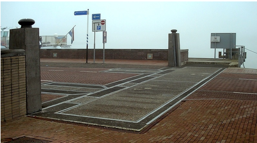
Figure A.15: Kampen: flap gate; the flood defence switches from the far side of the road (which is at the river side) to the near side, November 2011
