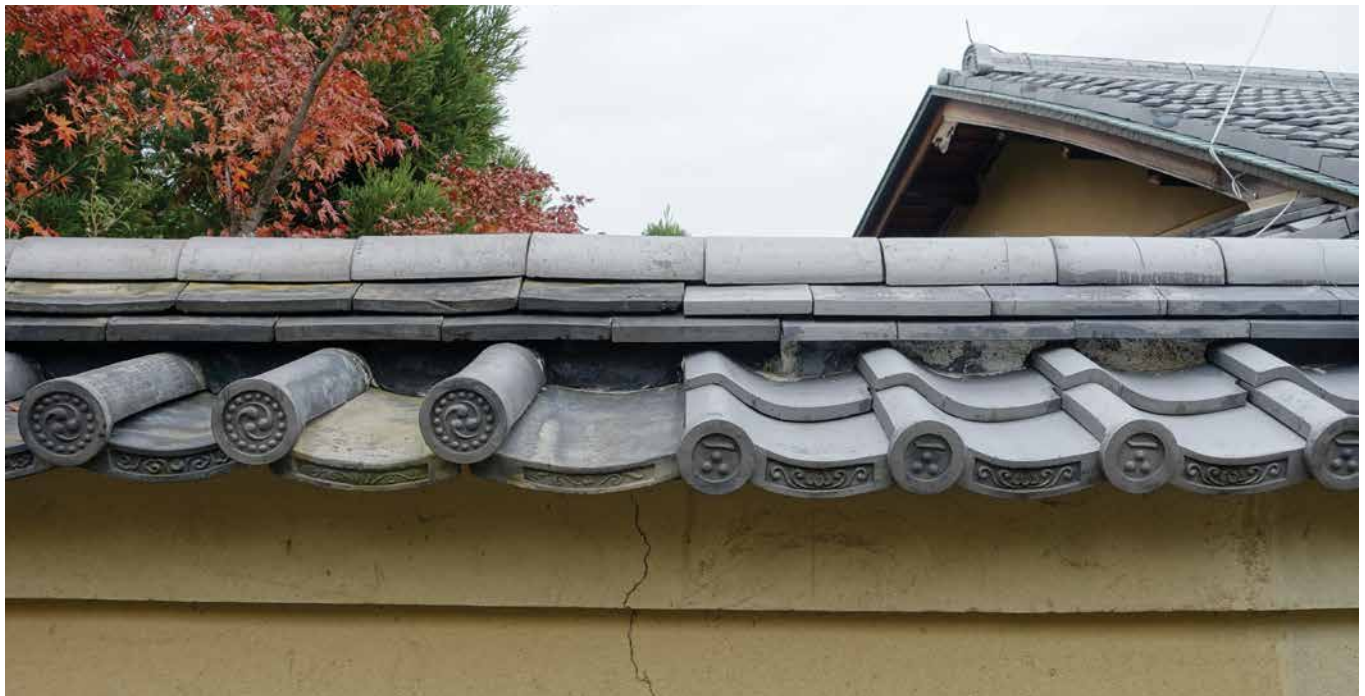
FIG. 19 Daitoku-Ji temple restored by Takamura with old and new tiles
