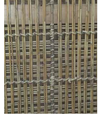
FIG. 4 Wooden frame with bamboo lattice bound by rice ropes on which the first, inner layer, of the earth wall has been applied (left). Wooden frame with reed lattice, before the application of the earth plaster (right)
