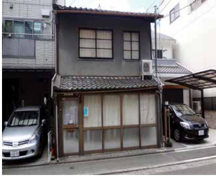
FIG. 3 Machiya before renovation
