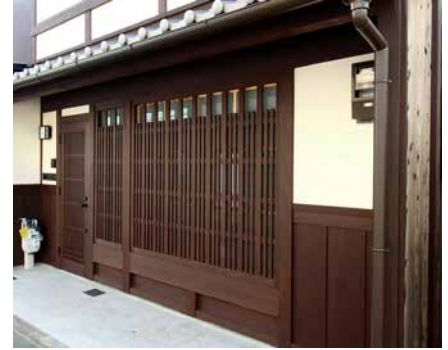
FIG. 5 Machiya after renovation
