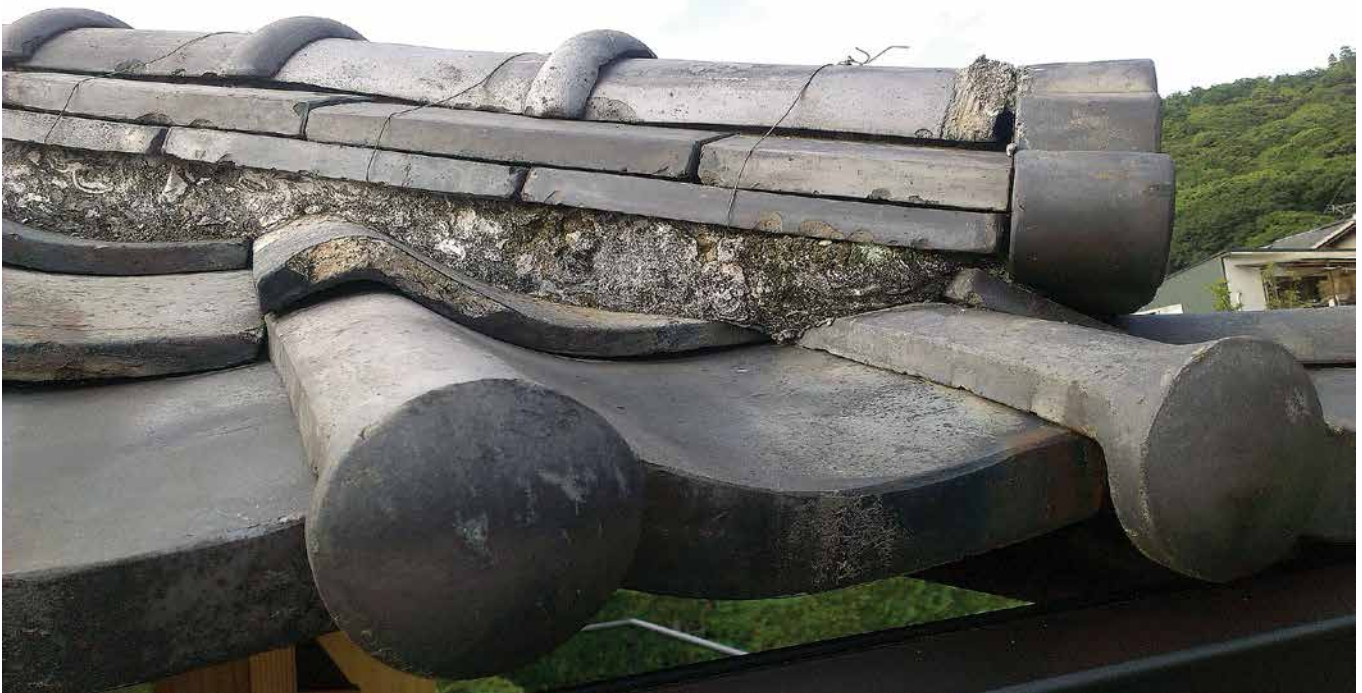
FIG. 19 The ridge of a roof in a recently restored machiya: roof tiles are laid on a bed of clay, lime and straw
