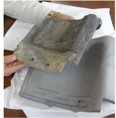
FIG. 15 Old and new roof tile
