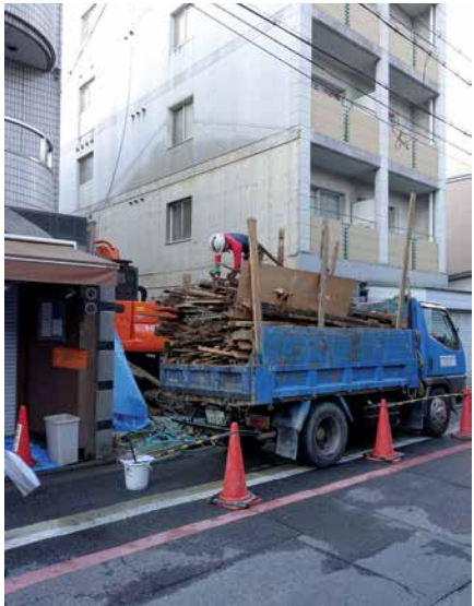
FIG. 18 A machiya pulled down and deported (2015)
