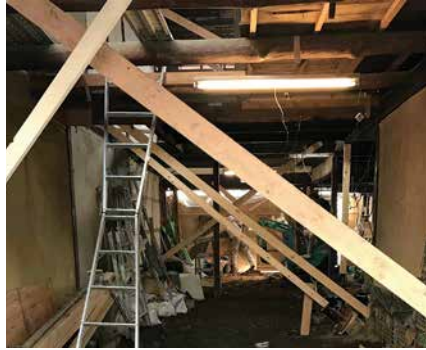
FIG. 4 Machiya under renovation
