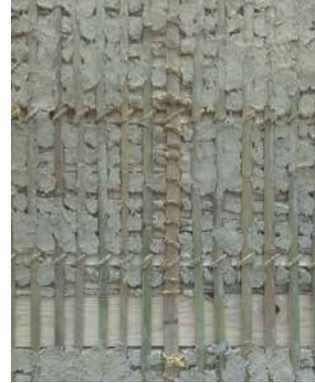
FIG. 4 Wooden frame with bamboo lattice bound by rice ropes on which the first, inner layer, of the earth wall has been applied (left). Wooden frame with reed lattice, before the application of the earth plaster (right)
