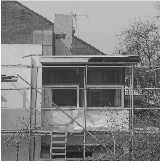
FIG. 1.7 The roof required extensive repairs to prevent further sagging and leaks
