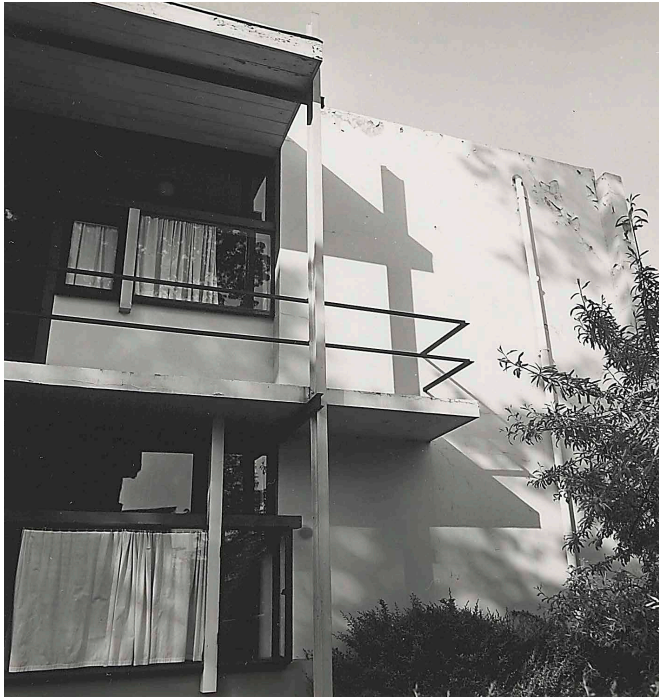
FIG. 1.2 Damage to the house became increasingly visible
