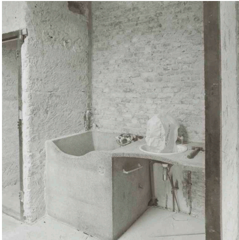
FIG. 3.7 Stripped bathroom with 'lavette'
