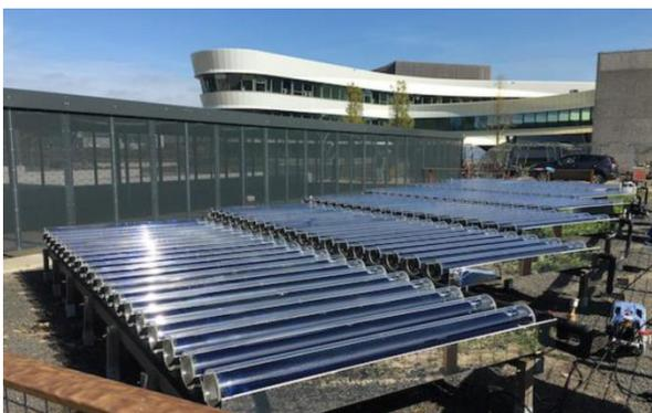
**Figure 7: Installed Virtu® PVT panels at Delft pilot site.**
