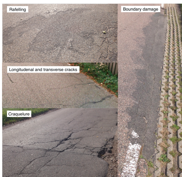
Figure 1. Examples of road surface damage.
