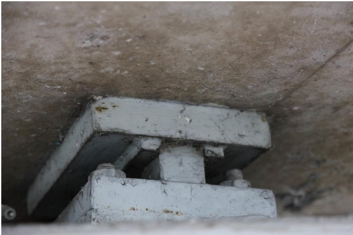
Figure 1. Example of frozen bearing.
