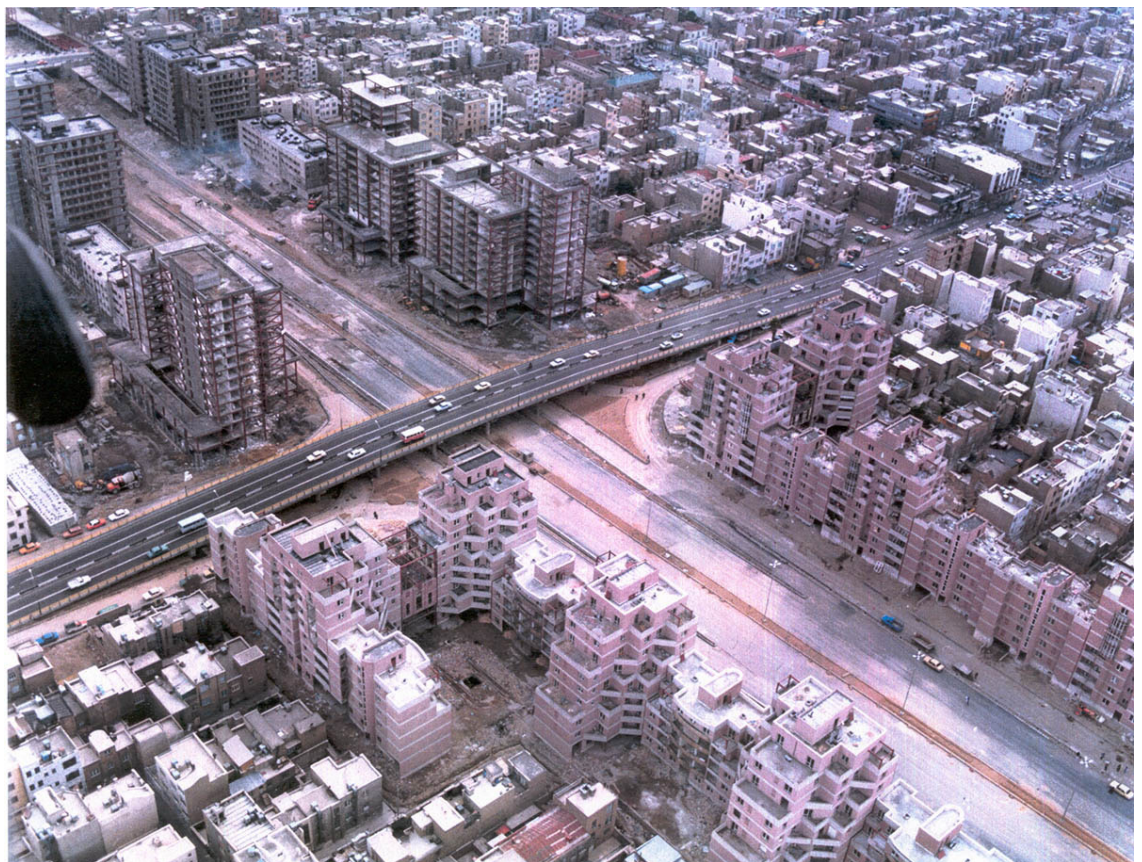
Figure. 5.9. Navab Residential Complex and Highway under construction
