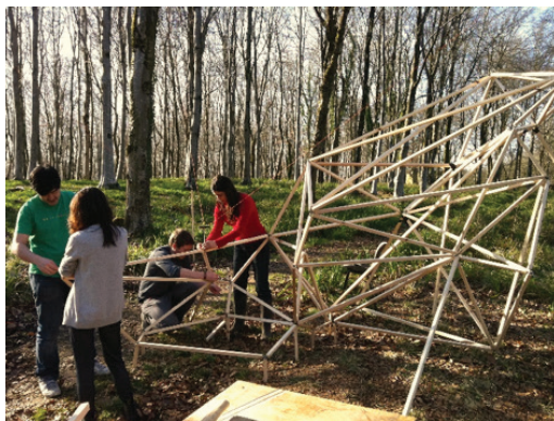
FIGURE 4 Human collaborators installing timber elements guided by the cable robot pointer, resulting in a variable density triangulated structure.
